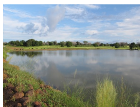
Irrigation dam in Tanchera
